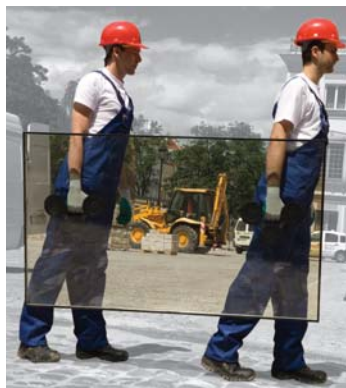
■ Manual grabs and suction caps can be used for relocating smaller objects.
