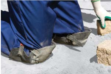
■ Protection of knees while paving.
