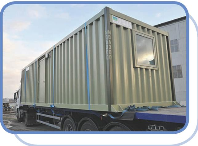
Figure 9. Typical site cabin based on ISO Container footprint
