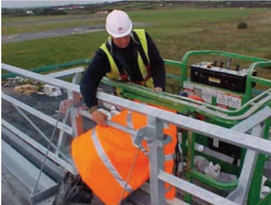
Figure 9.1: Access point to roof convenient to working position.
