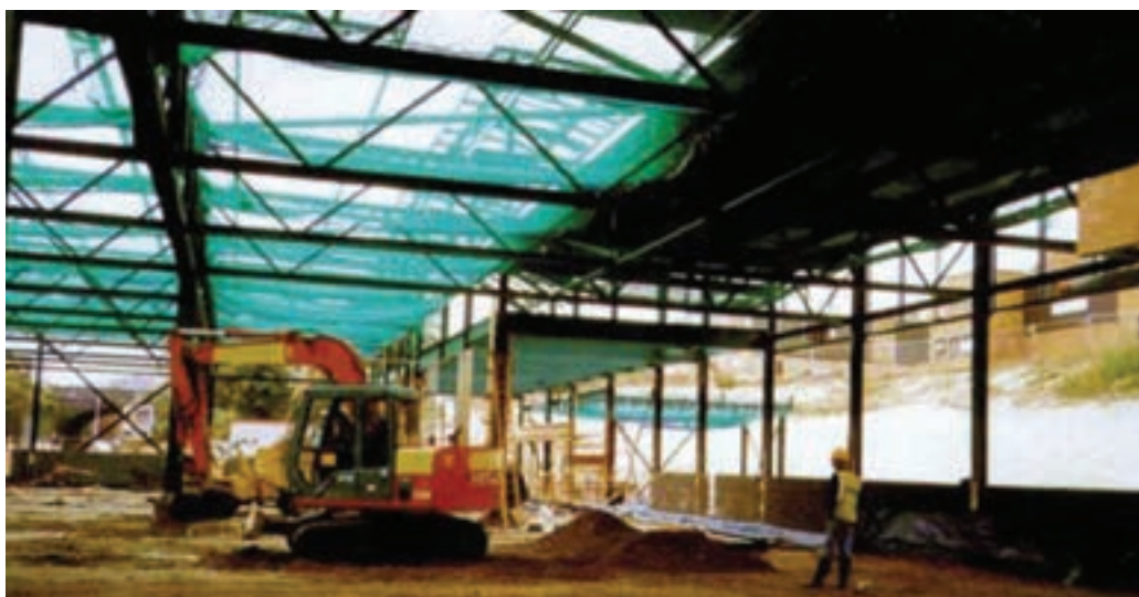
Figure 11.4: Debris netting in addition to safety netting may enable work to be carried out safely below roof workers
