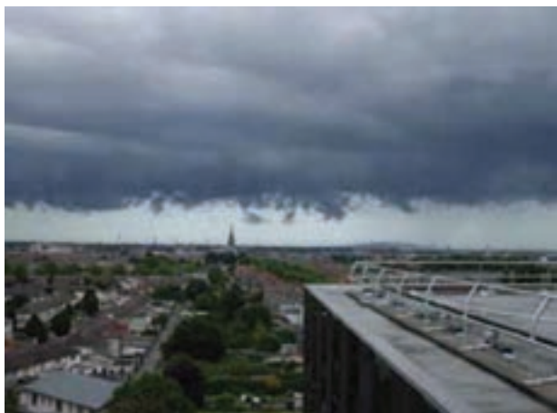
Figure 4.5: Permanent guard-rails retrofitted during refurbishment work. Similar protection can be included during initial designs.
