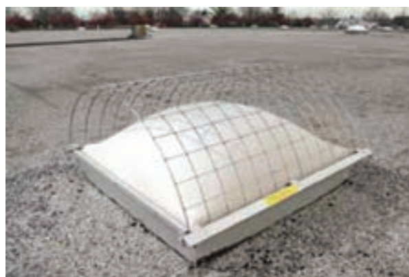
Figure 4.8: (a) Galvanised mesh reinforcement between sheets of twin skinned rooflight and (b) guard-rail fitted over a rooflight.
