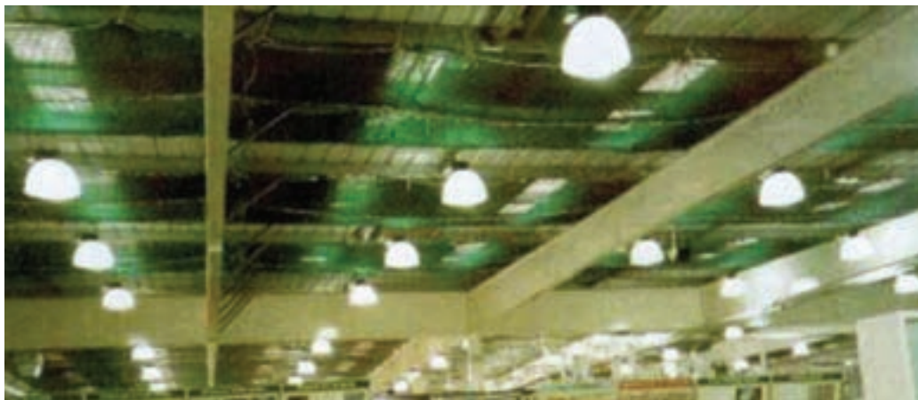
Figure 9.8: Safety netting providing protection for rooflights during minor roofwork.
