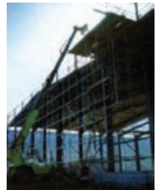
Figure 9.2(a): Delivery of sheets to roof level onto the completed load-bearing section and behind the leading edge. (Note the rooflights include mesh protection rendering the assembly non-fragile.)
