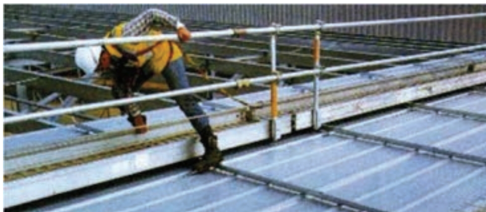
Figure 9.4: Trolleys can sometimes become difficult to move which can force operators into dangerous positions
