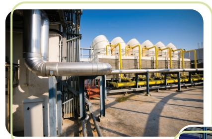
They are found in many different places of work from food or pharmaceutical processing plants to hotels or offices. Towers can have an open or closed circuit or a combination of both, they can be either induced or forced draught type, with a counter or cross-flow of air relative to the water flow.
