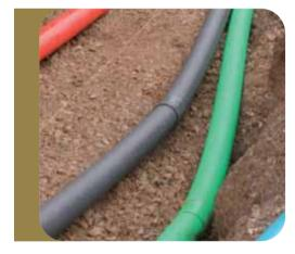
Telecommunications cables may be installed in concrete pipes, smooth black ducting or grey corrugated ducting. All cables should be assumed to be live until disconnected and proved to be safe. Contractors should obtain written confirmation of disconnection from the utility/service provider before removing a redundant service or arrange for the utility/service provider to remove the service.
