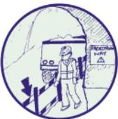
Whether workers on site or members of the public accessing close to demolition works, separating pedestrians from construction and demolition plant operations is important. Dedicated pedestrian routes clearly identified must be used.
