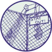
There should be a designated area fenced area for parking vehicles and storing materials. There should be a safe pedestrian walkway clearly marked out. At the end of the day the compound must be secured to prevent unauthorised access.
