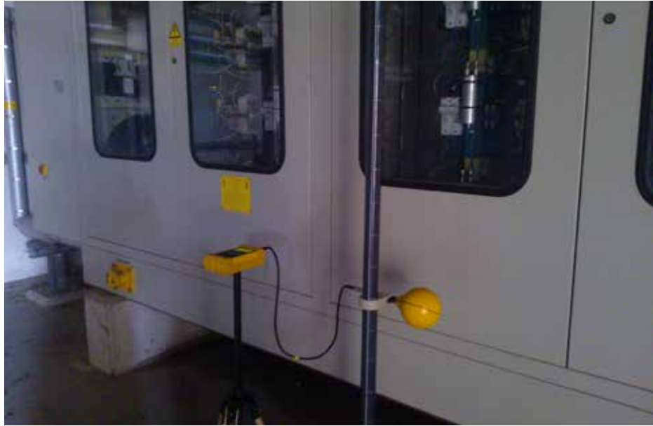
Figure 3.6 — Measurements being made near a thyristor rectifier
