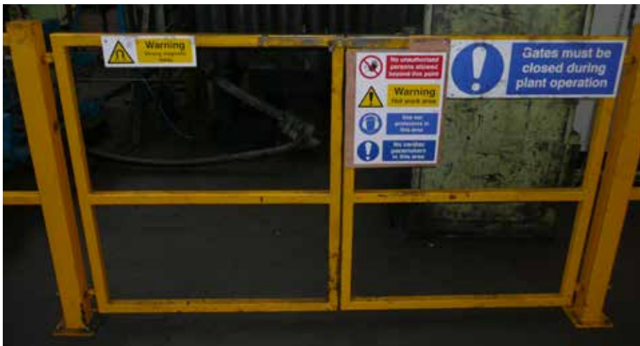
Figure 9.1 — Example of a simple moveable guard used to restrict access to a strong magnetic field. In this case the guard is not interlocked, but is supplemented by warning signs and organisational measures
