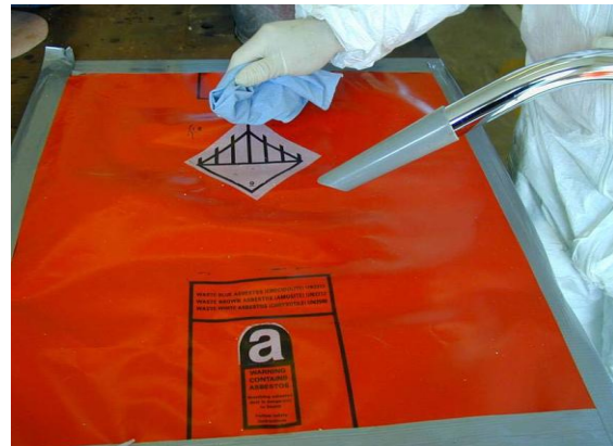
Cleaning up the work area carefully, with H-Type vacuum cleaner and wet waste rags.
