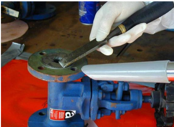
Use of shadow vacuuming to capture dust released in cleaning asbestos from a valve.
