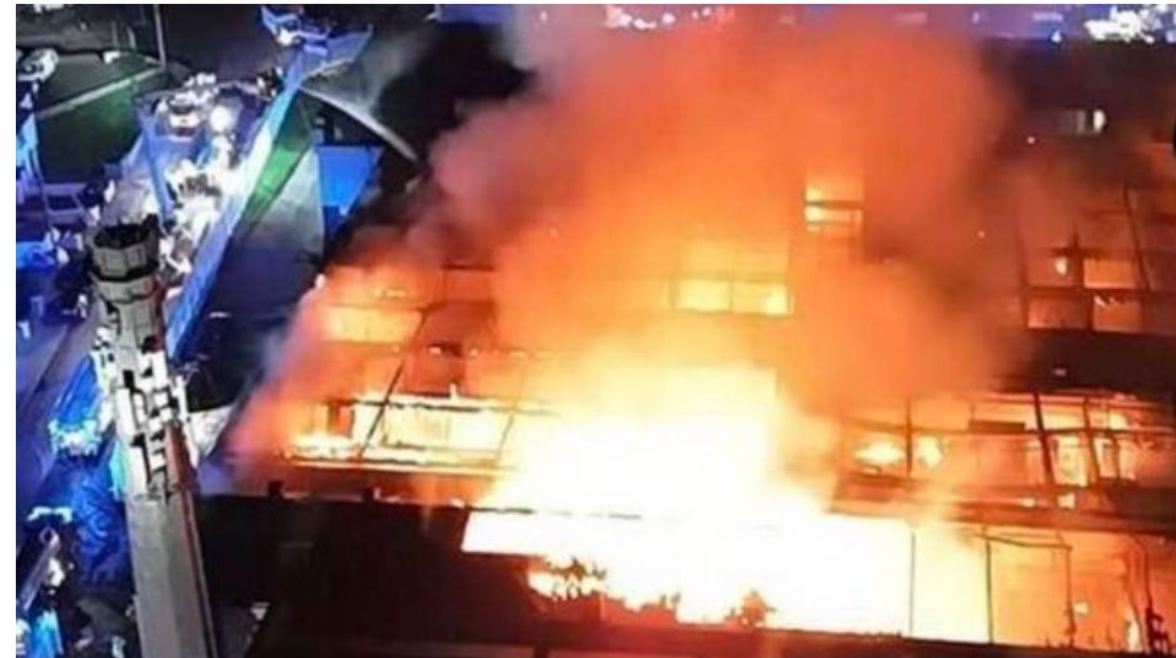
Fire at a Tycor Business Park, Waterford 09-May-2026
